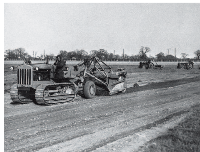
Levelling the site for the new grass airfield at Burnaston, April 1938.
